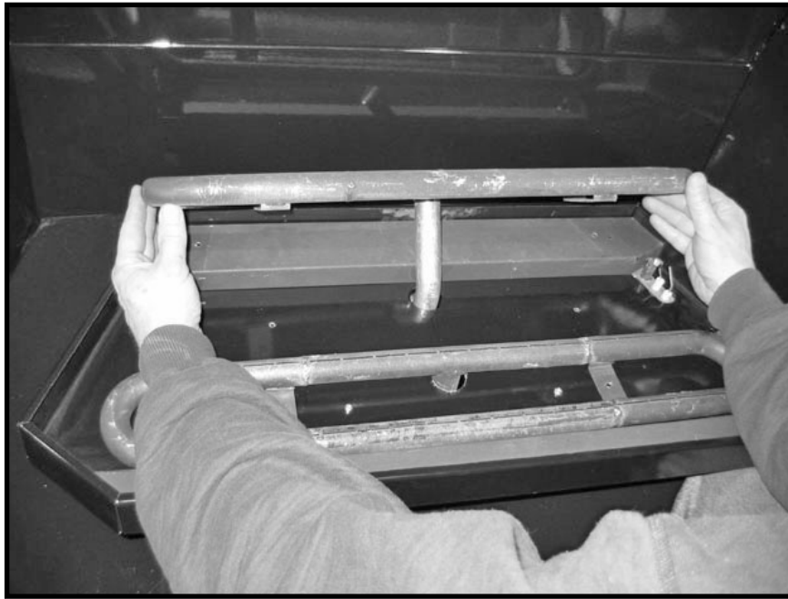
Figure 17: Install Rear burner.
