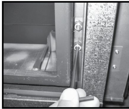
Figure 21: Gas pressure adjustment location.
