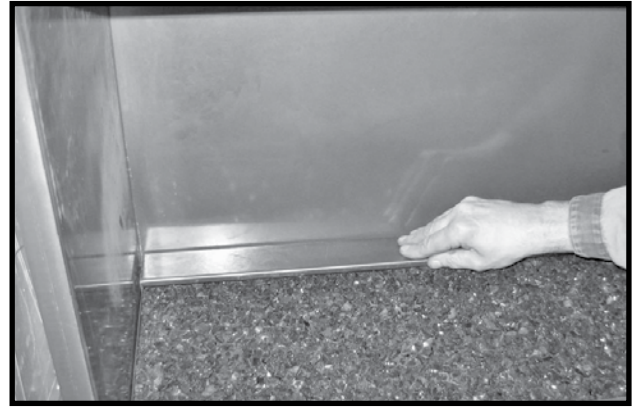
Figure 9: Placing rear trim.
