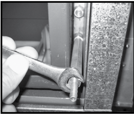
Figure 20: Gas pressure adjustment fitting.
