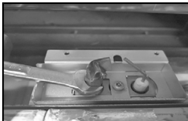
Figure 15: Loosening the pilot.
