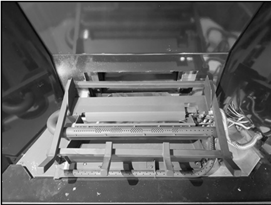
Figure 24: Burner and log grate installed.
