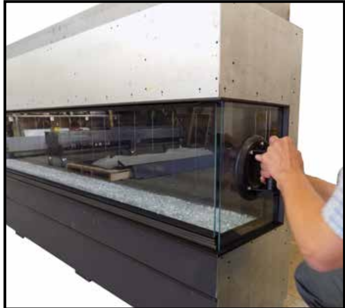
Figure 50: Lowering outside right hand side plate.
