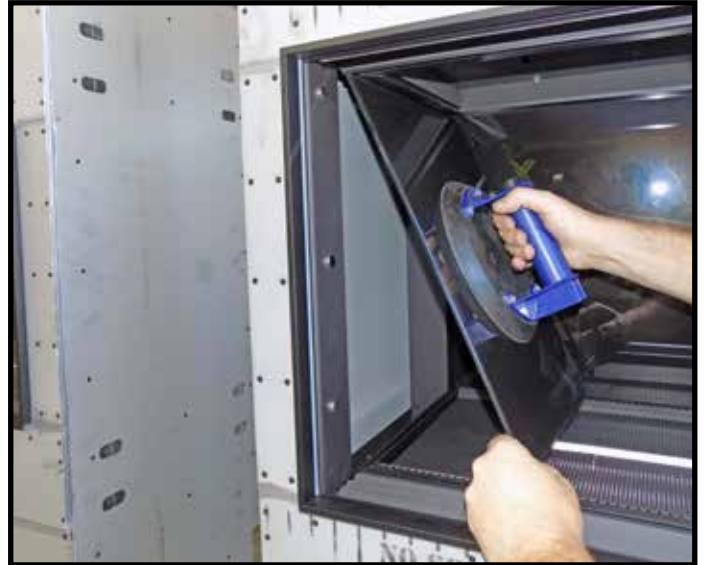
Figure 37: Insert top of side black glass first.
