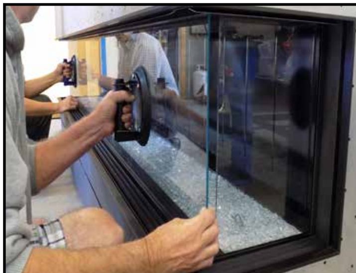
Figure 51: Installing the inside front glass plate.
