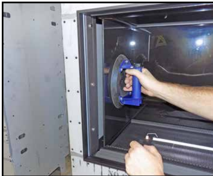
Figure 38: Insert bottom end of side black glass plate.
