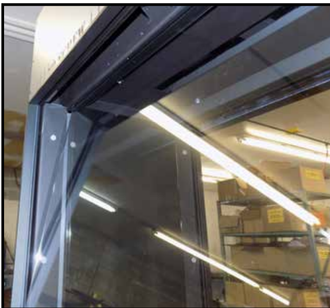
Figure 45: Top edge of sheet goes in first.
