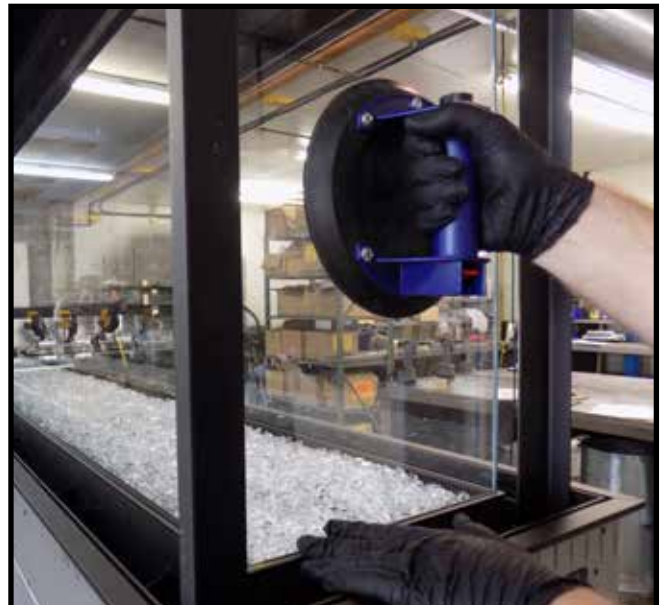
Figure 46: Installing inner end glass sheet.
