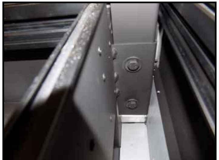
Figure 10: Lower support bolts to be removed.
