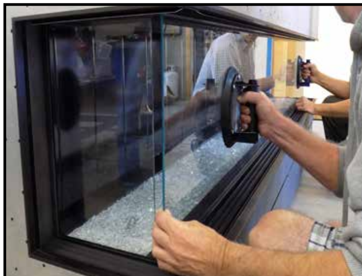
Figure 49: Installing the inside front glass plate.
