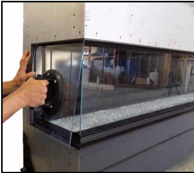
Figure 47: Installing outside right hand side plate.
