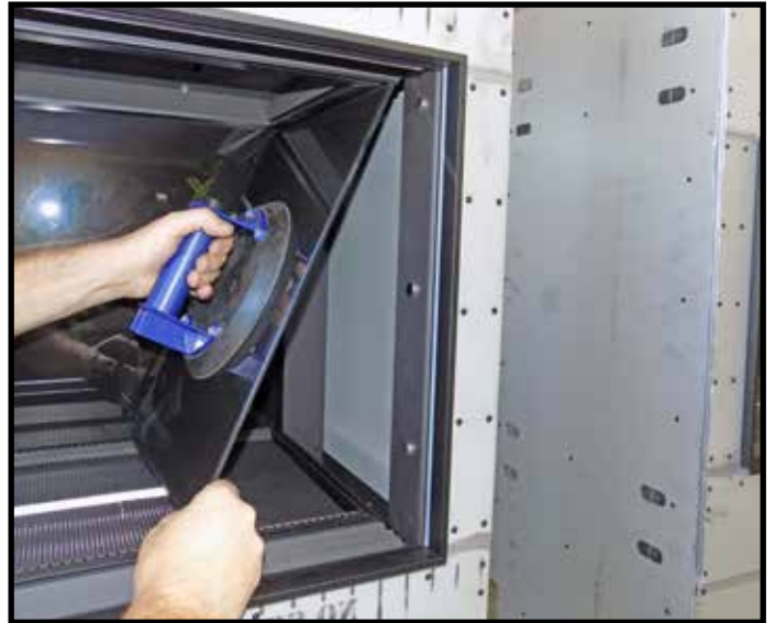
Figure 35: Insert top of side black glass first.
