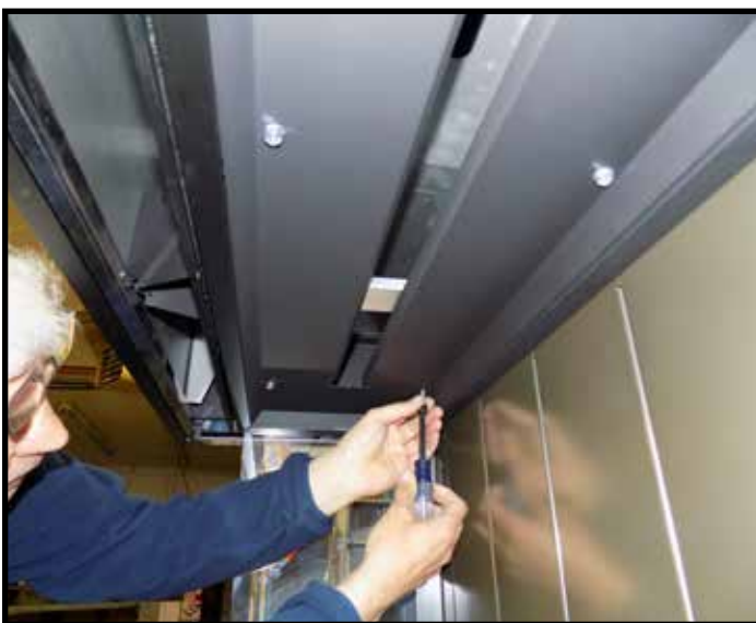
Figure 27: Securing the baffle cover.
