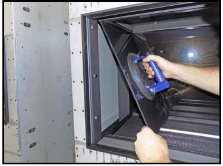
Figure 30: Insert top of side black glass first.
