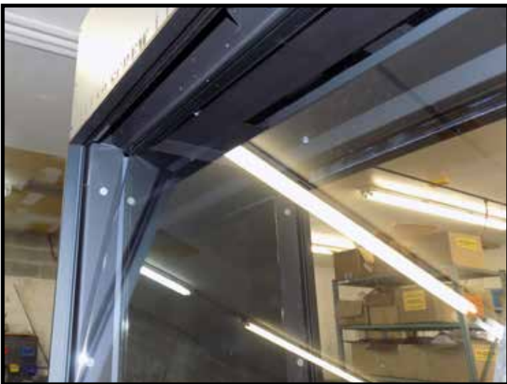
Figure 37: Top edge of sheet goes in first.
