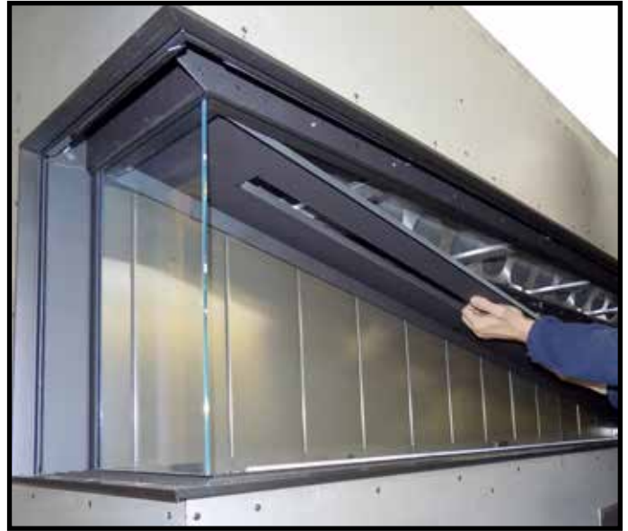
Figure 26: Installing baffle cover.
