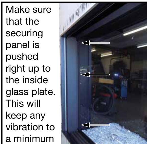
Figure 41: Position securing panel up against the inside glass plate.
