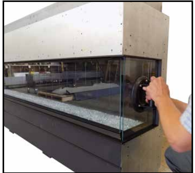
Figure 53: Installing outside right hand side plate.
