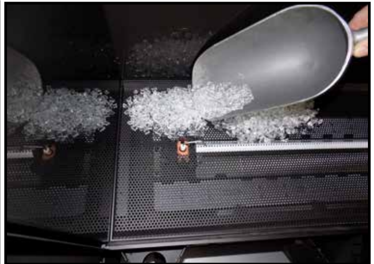
Figure 41: Applying crushed glass on burner tray.
