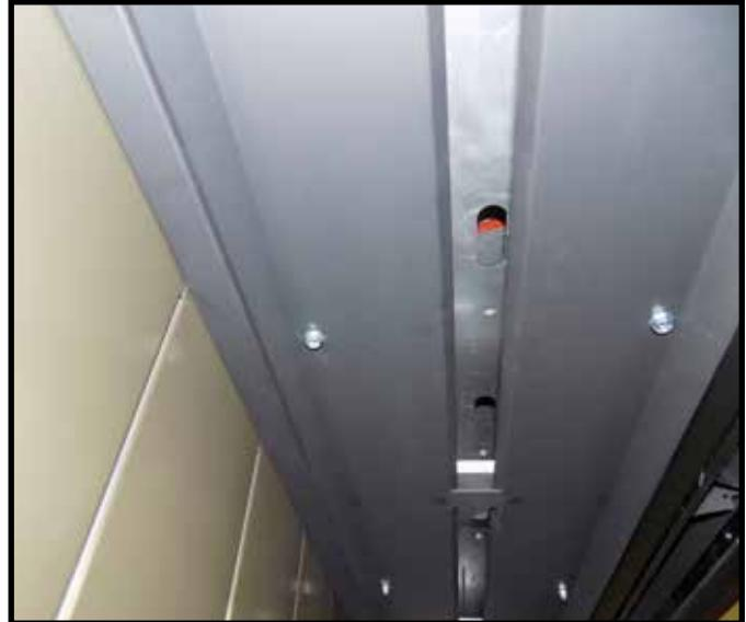
Figure 29: Adjustment accessible through the baffle cover.
