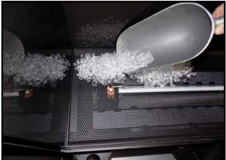
Figure 41: Applying crushed glass on burner tray.
