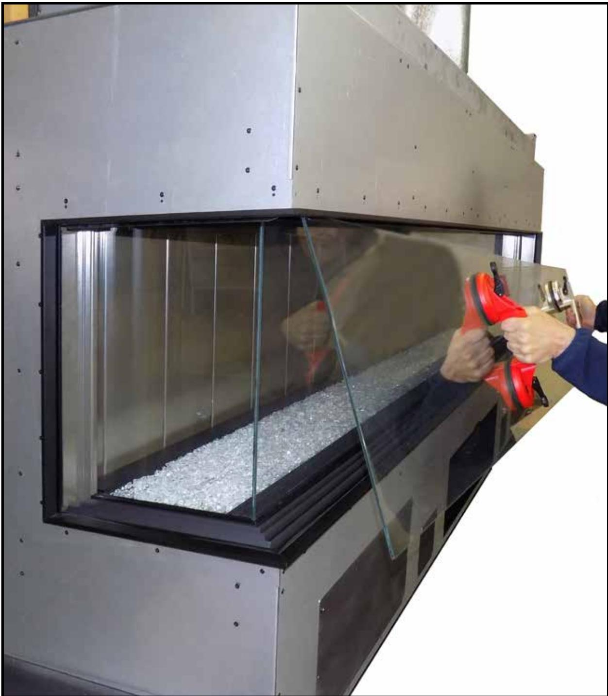
Figure 54: Inserting top edge of outside front plate.
