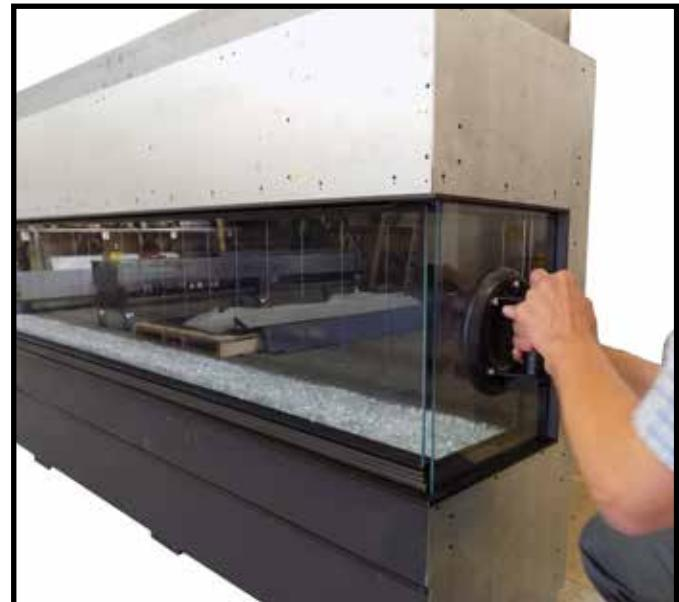
Figure 53: Installing outside right hand side plate.
