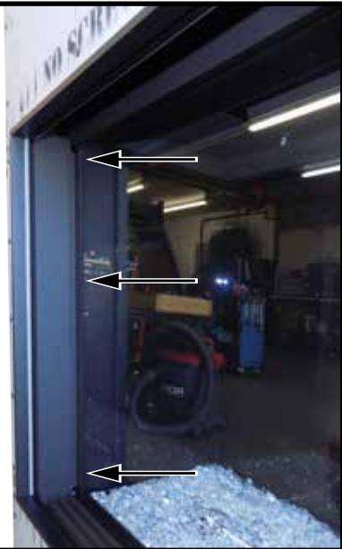
Figure 50: Position securing panel up against the inside glass plate.
