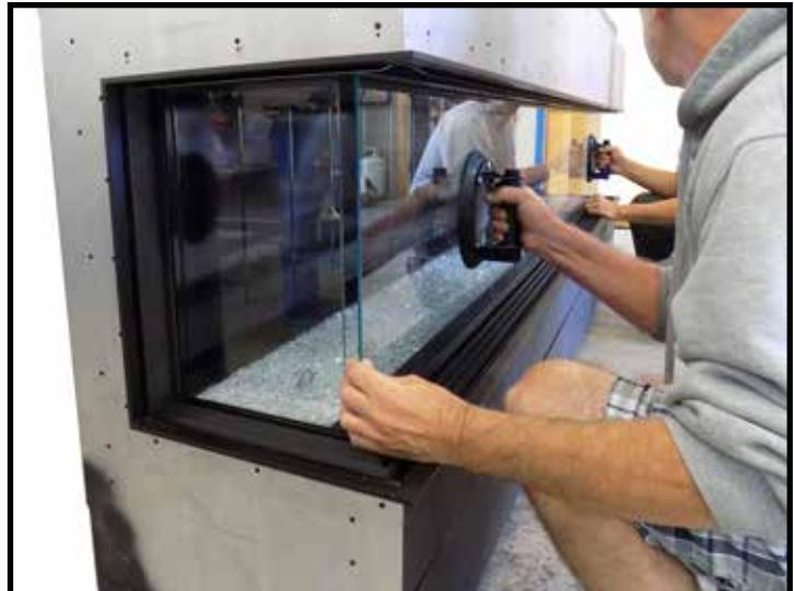
Figure 45: Installing the inside front glass plate.
