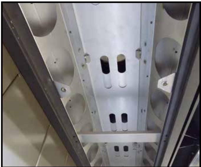
Figure 28: Adjustable baffle ports.
