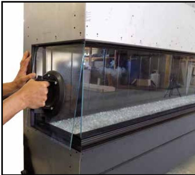
Figure 52: Installing outside left hand side plate.
