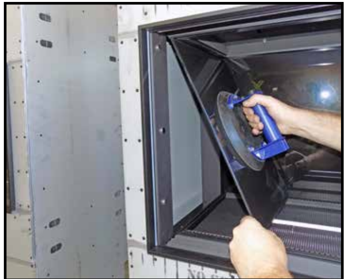
Figure 36: Insert top of side black glass first.
