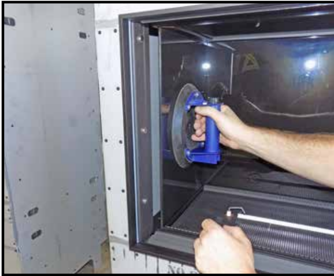
Figure 37: Insert bottom end of side black glass plate.
