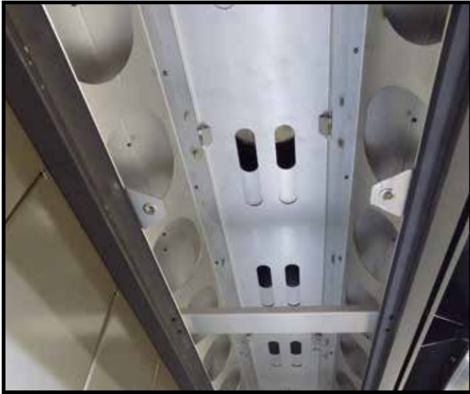
Figure 30: Adjustable baffle ports.
