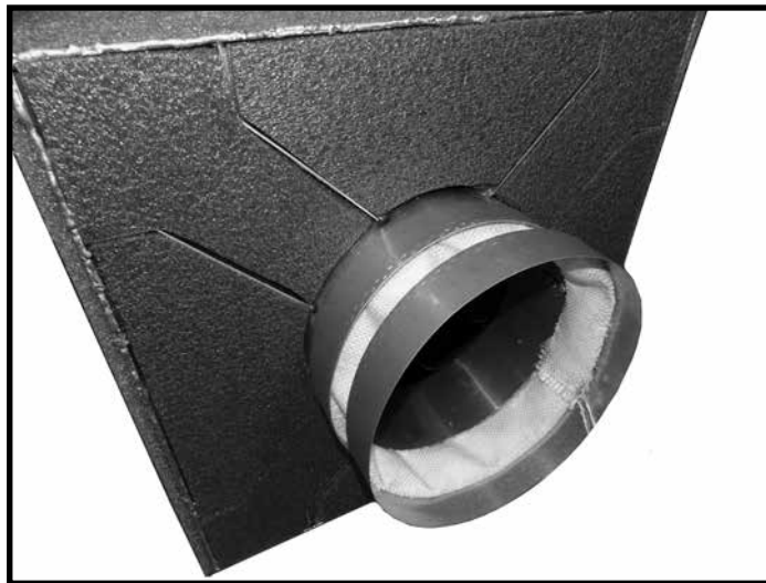
Figure 12: Vibration collar installed.
