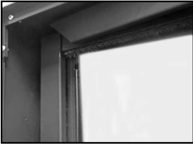
Figure 67: Installing top trim.
