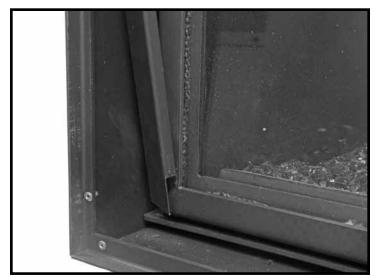
Figure 55: Installing the side trim.
