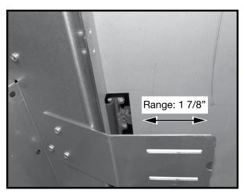
Figure 20: Framing bracket.
