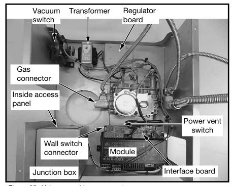
Figure 25: Valve assembly components.
