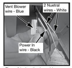
Figure 24: Junction box wiring.
