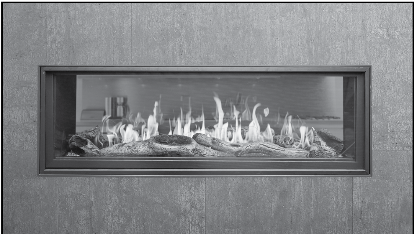
Figure 26: Example of desirable flame pattern.
