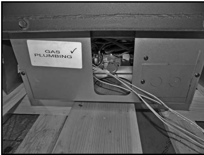
Figure 5: Lights wiring coming from grommet.
