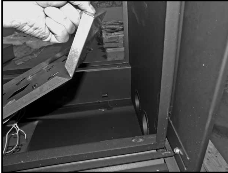
Figure 1: Inserting secondary floor panel into the right side.
