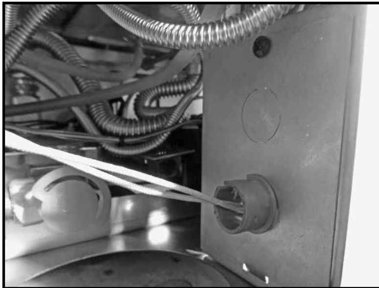
Figure 6: Threading wires through knockout.
