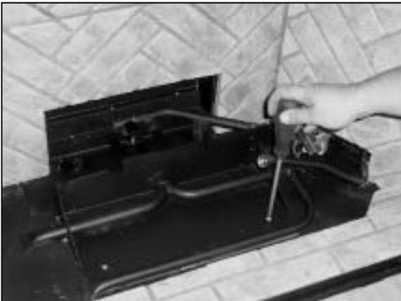
1. Attach the burner assembly to the bottom of the firebox with two screws (Fig. #1).
