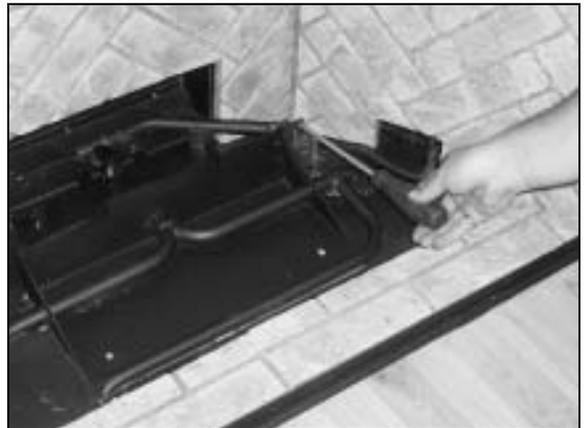
2. Attach pilot bracket to burner assembly (Fig. #2).
