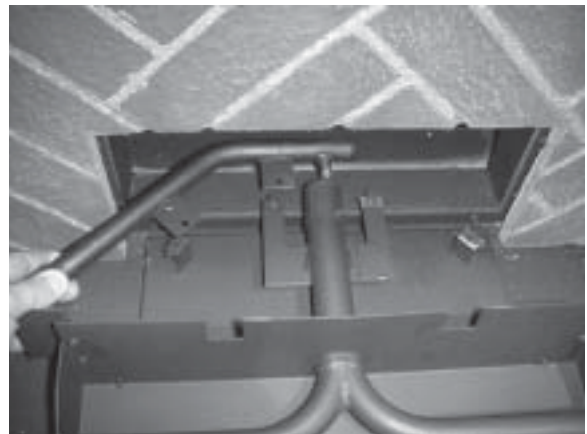
REPOSITION MANIFOLD
