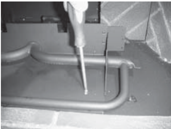
BURNER TRAY INSTALLATION
