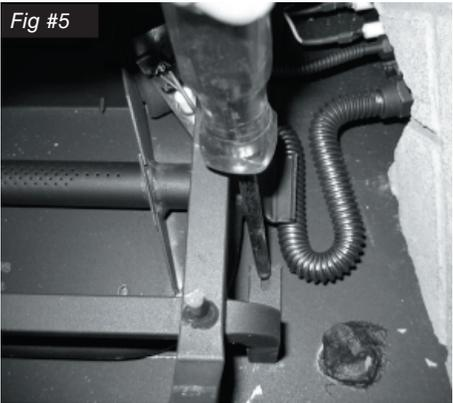
5. Position the grate over the burner tray and attach to the floor with two screws through holes located behind the front legs of the grate. (Fig. # 5)
