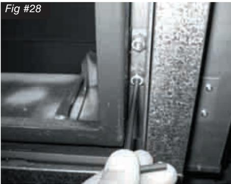
1. Remove the blanking plug from the pressure test port. The plug is located between the right side lintel and firebox side. (Fig. #28)
