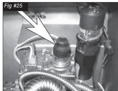
14. Press down on the center post and rotate 90°. The center post should stay down. (Fig. #26). Replace the rubber cap.
