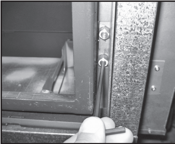
Figure 42: Removing manifold pressure plug.
