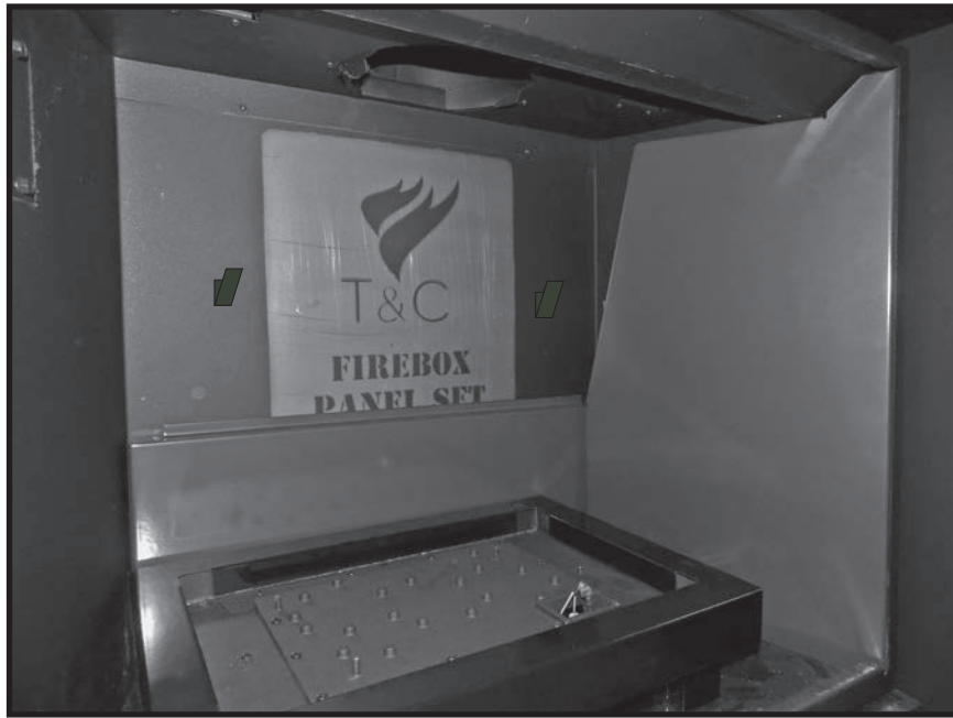
Figure 18: Right side panel partially installed.
