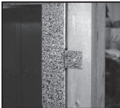
Figure 18: Attaching metal tab to frame.
