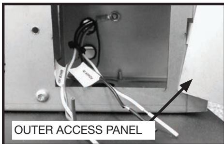
Figure 25: Junction box wiring.
