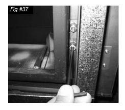
Remove the plug from the pressure test port using a 3/16" hex key. The plug is located between the right side lintel and firebox side. (Fig. #37)
