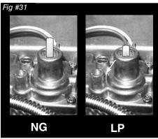
Press down on the center post and rotate 90°. The center post should stay down. (Fig. #31). Replace the aluminum cap.
