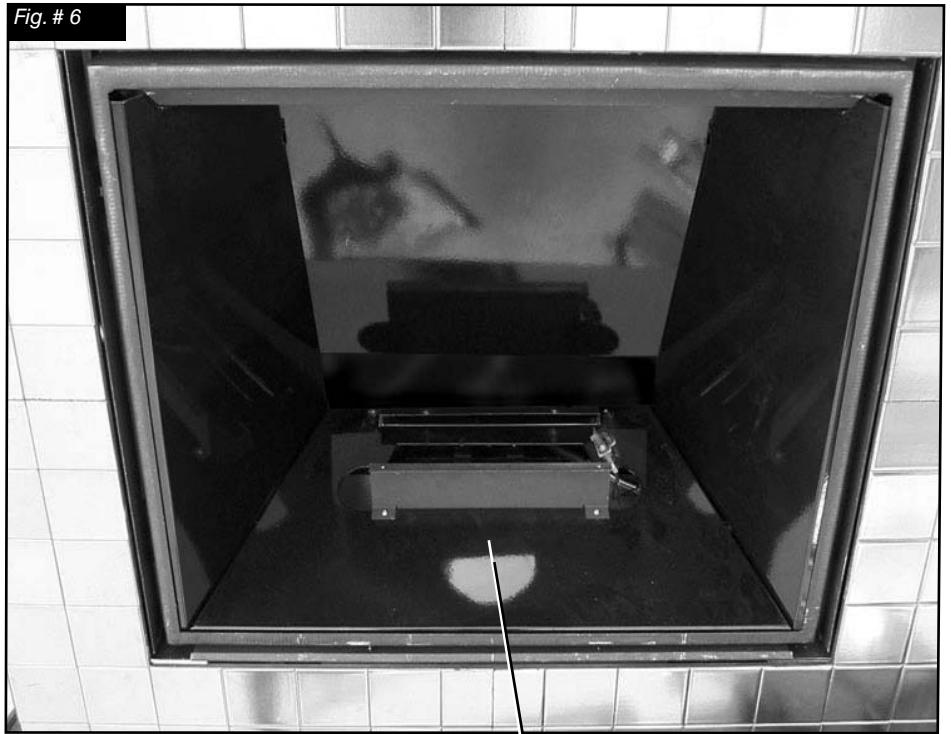
INSTALLING BURNER SHIELD
